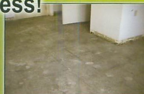
Ready to Resurface!
